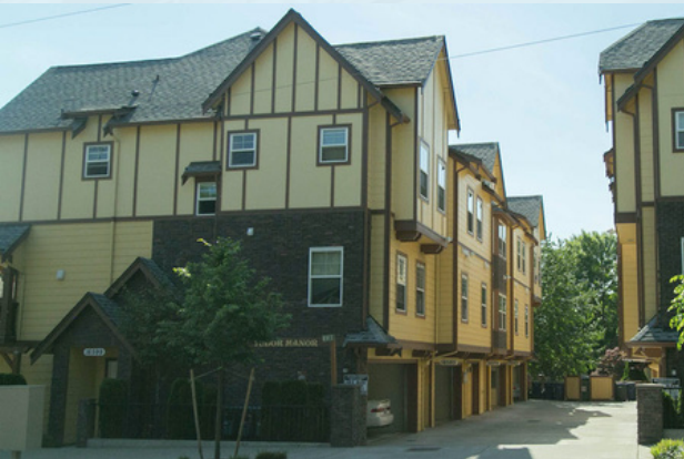
Tudor Apartments, a 61-unit co-living development in Redmond developed by Natural and Built Environments
